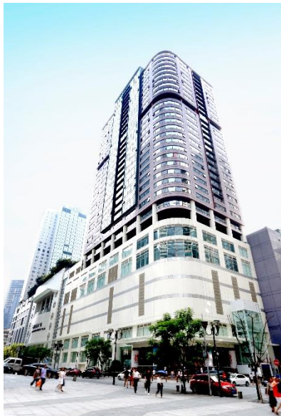
The Tower at Chongqing Metropolitan Oriental Plaza
